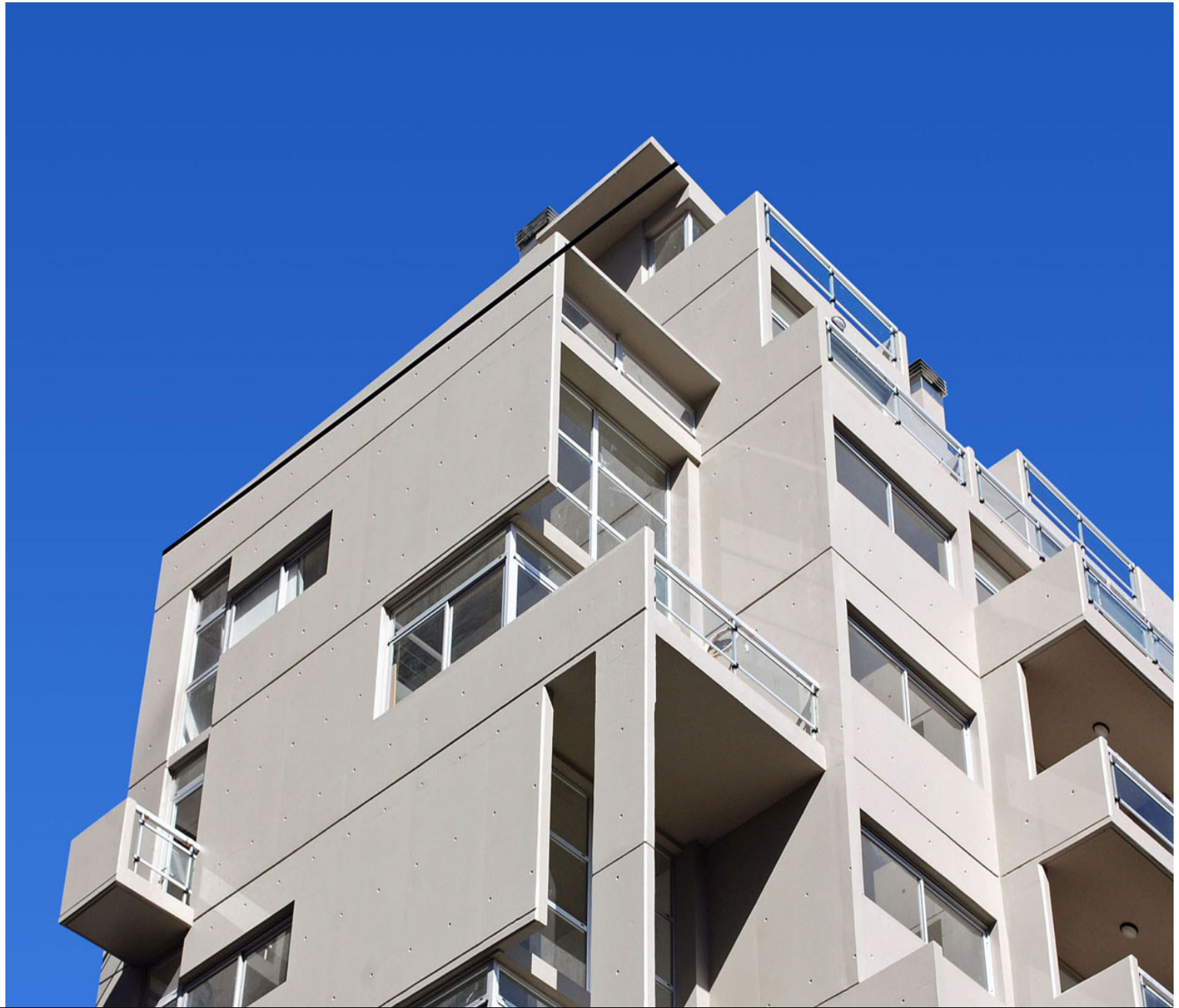
Balconies and upper terraces Modelle Plaza Building, Buenos Aires, Argentina
