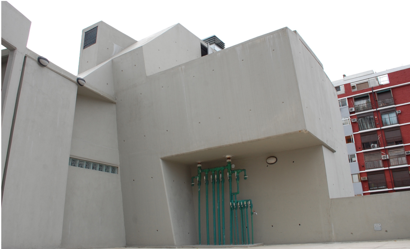
View of the building's water tank Modelle Plaza Building, Buenos Aires, Argentina
